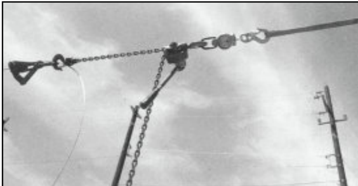
A-20S with top hoist hook in Campbell link.
