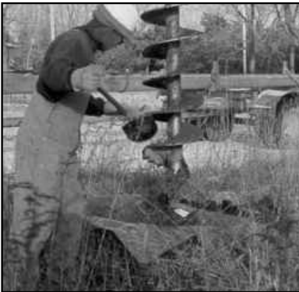
Cleaning auger onto TWISTARP.
