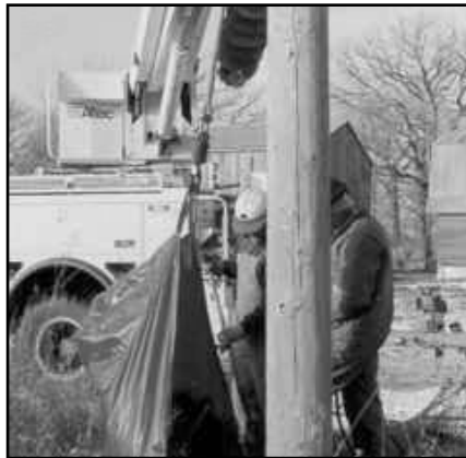
Winch dirt out of weeds. Trucks help put dirt back in hole. Tarp does not hinder tamping.
