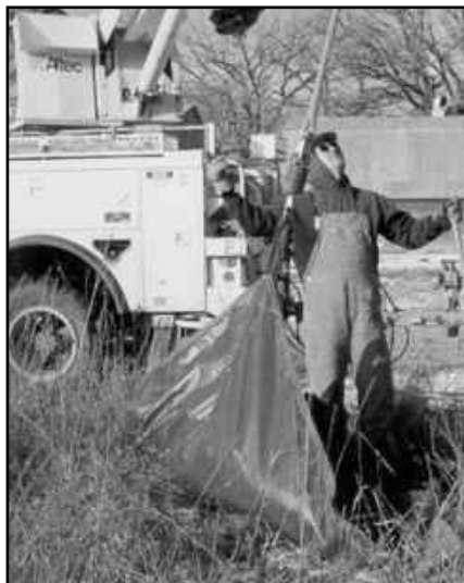
Winching TWISTARP with truck for filling.
