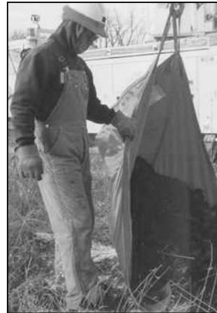
Dumping TWISTARP with winch to fill hole.
