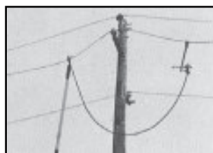
Install other end of jumper on conductor.
